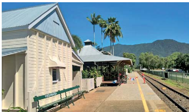
Upgrade at Queensland Rail's Freshwater Station in Far North Queensland.
