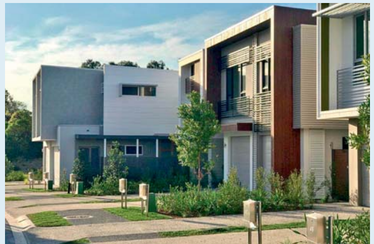
Hutchies is currently completing construction of 54 three-bedroom, two-storey townhouses at Robina's City Village.
