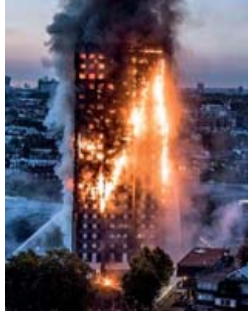
The Grenfell Tower tragedy in London sparked an international alert on combustible wall cladding.
